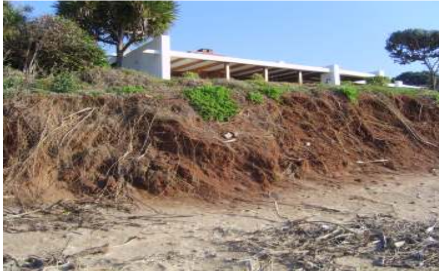
Plate 5.2: Damage to the dunes from the storms and subsequent waves
